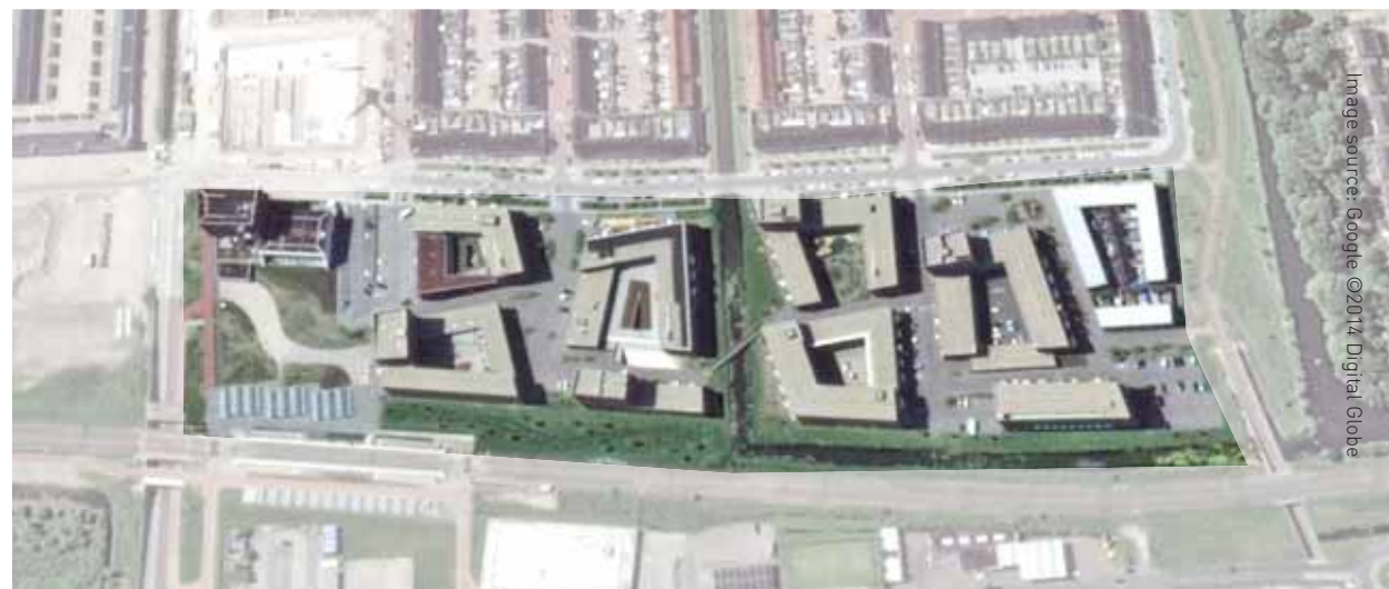
Located in the centre of Pijnacker, Weidevogelhof services the entire new community west of the train line with the intention of being a truly integrated health and housing precinct
